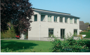
23 WOONHUIS WIM RAMSELAAR, CA. 1977 POLDERSTRAAT 22, MACHAREN [P.75 BOSSCHE SCHOOL IN OSS]
